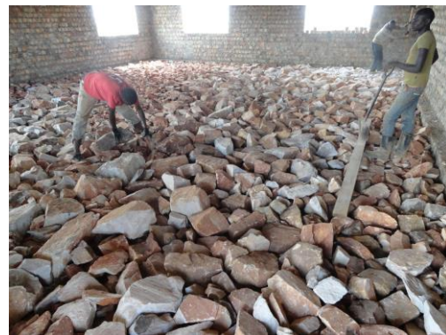
We started to bring in trips of stones (known as hard cored) to prepare the floor. The entire building needed tones and tones close to 30 trips to cover the floor. Men worked for many days ferrying the stones into the rooms and using sledge hammers to hit them into position. It was hard labor for them, but it was completed and the floor was now ready for concrete. We also spray chemicals at this stage to deal with termites which would otherwise remain active underneath the foundation.
