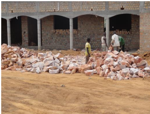
We started to bring in trips of stones (known as hard cored) to prepare the floor. The entire building needed tones and tones close to 30 trips to cover the floor. Men worked for many days ferrying the stones into the rooms and using sledge hammers to hit them into position. It was hard labor for them, but it was completed and the floor was now ready for concrete. We also spray chemicals at this stage to deal with termites which would otherwise remain active underneath the foundation.
