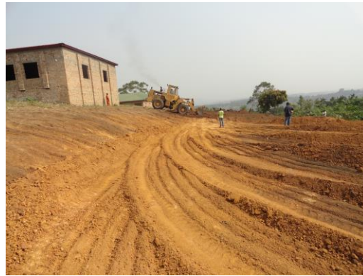
The final shape was after three days of work with the tractor (known as a wheel loader). It is hired per day at unique costs which are also influenced by scarcity of such equipment and the dear price of diesel
